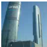
UAE, Abu Dhabi, Sun and Sky Towers Al Reem Island Luxury residential buildings Simplebus TOP and CCTV System 1104 Planux
